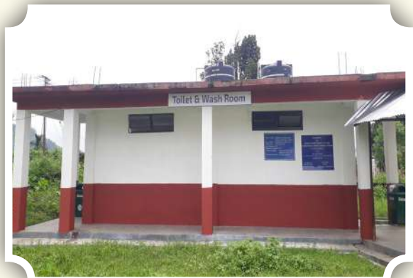
Common Toilet & Wash Room, DNGC, Itanagar
